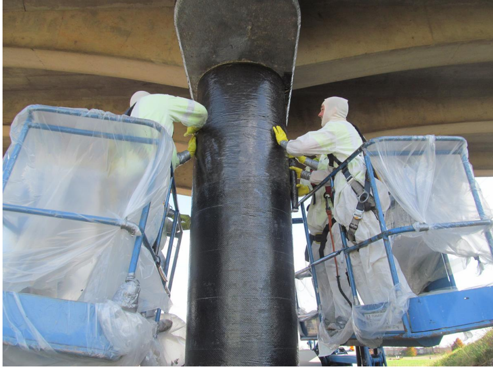
Figure 5.19 –Application of Triaxial Carbon Fabric
