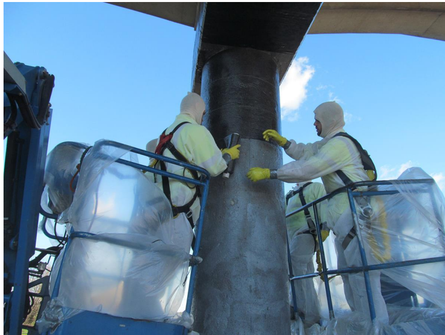
Figure 5.18 – Application of Unidirectional Carbon Fabric
