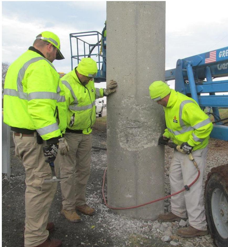
Figure 5.15 – Removing loose concrete material
