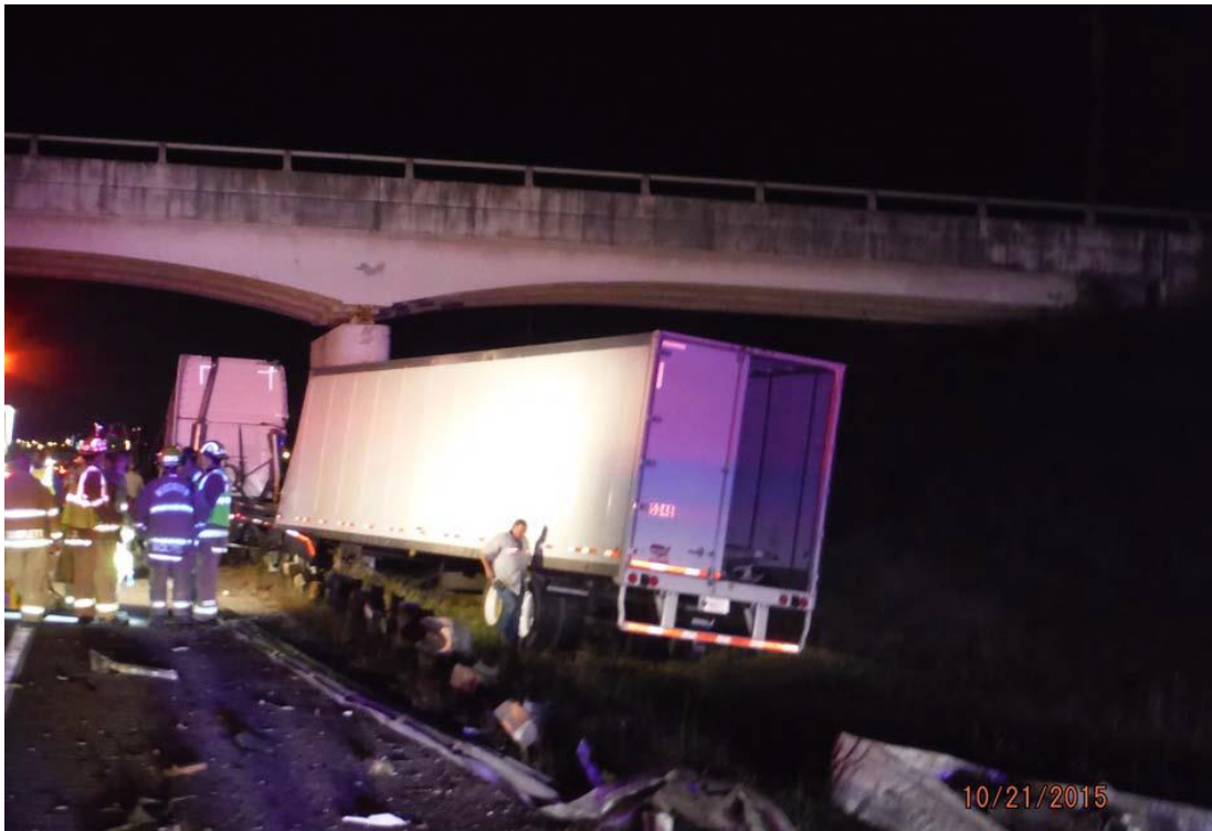
Figure 5.12 – Unloaded Semi Trailer that Impacted the Bridge Pier
