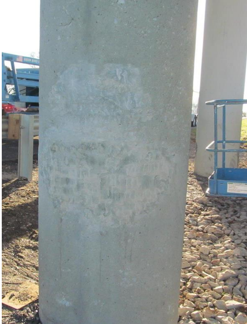
Figure 5.16 – Placement of repair mortar
